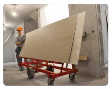
The Transit Bench as a stable workbench to enable easy and precise cutting of plasterboard.
